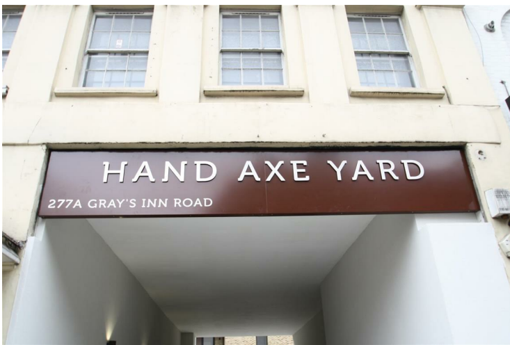
GRAYS INN ROAD ENTRANCE
