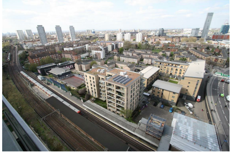
VIEW OF BROMLEY BY BOW STATION
